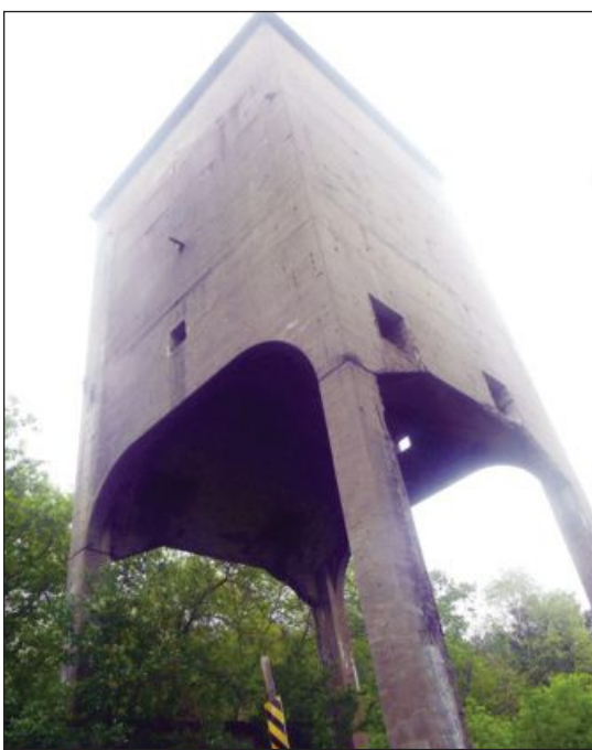
The old coal tower in Lake is shown from below. The adjacent bike path affords an opportunity for up-close viewing of the historical site.
